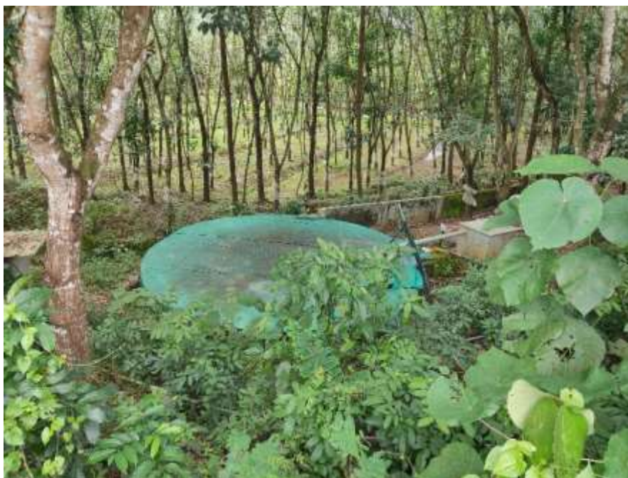
FIGURE 12 GROUND WATER RECHARGING WELL
